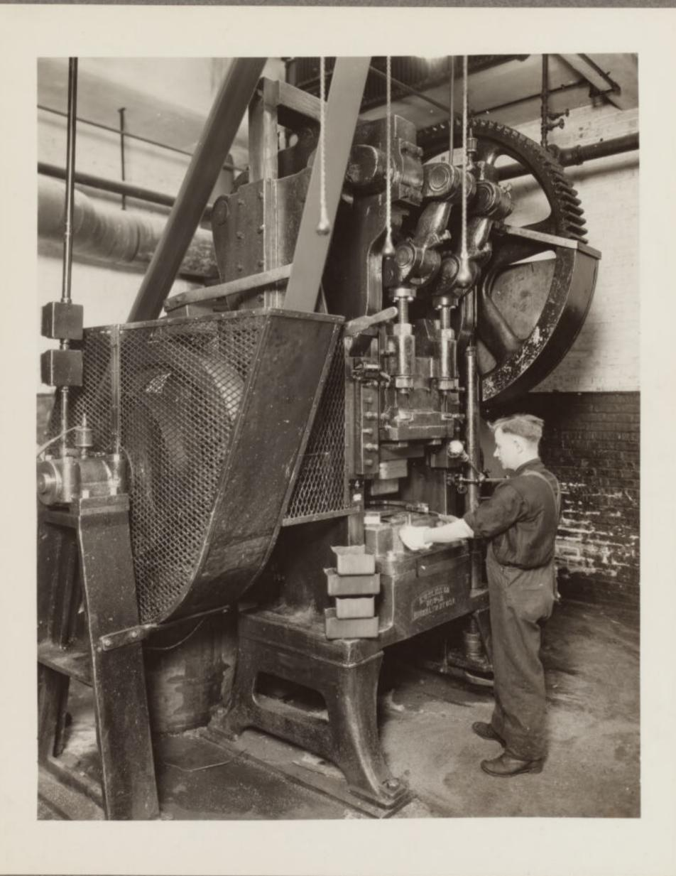
DOUBLE ACTION BLANKING AND DRAWING PRESS FOR SUBSCRIBER SET HOUSINGS
