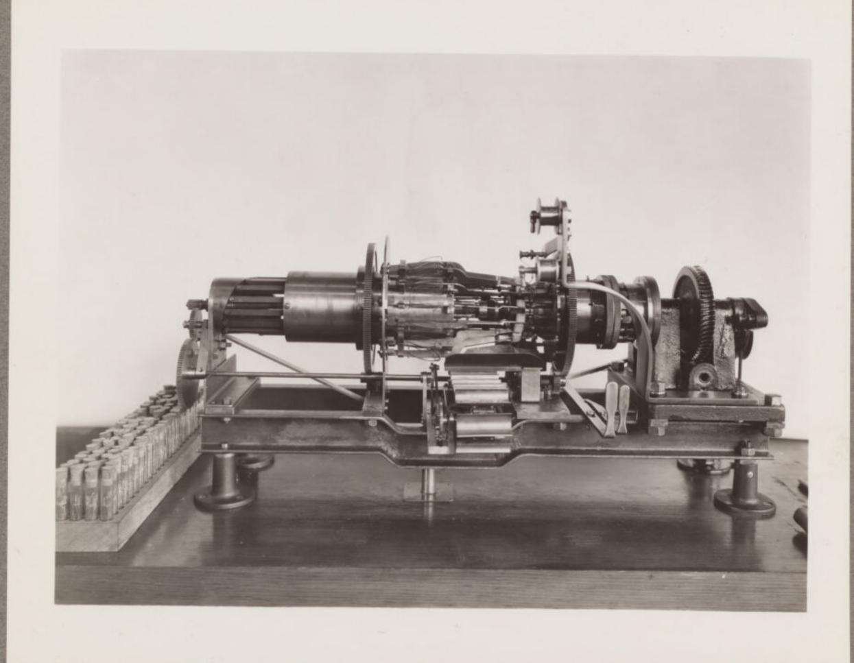
SWITCHBOARD LAMP LEAD-IN AND MOUNT WIRE WELDING MACHINE
