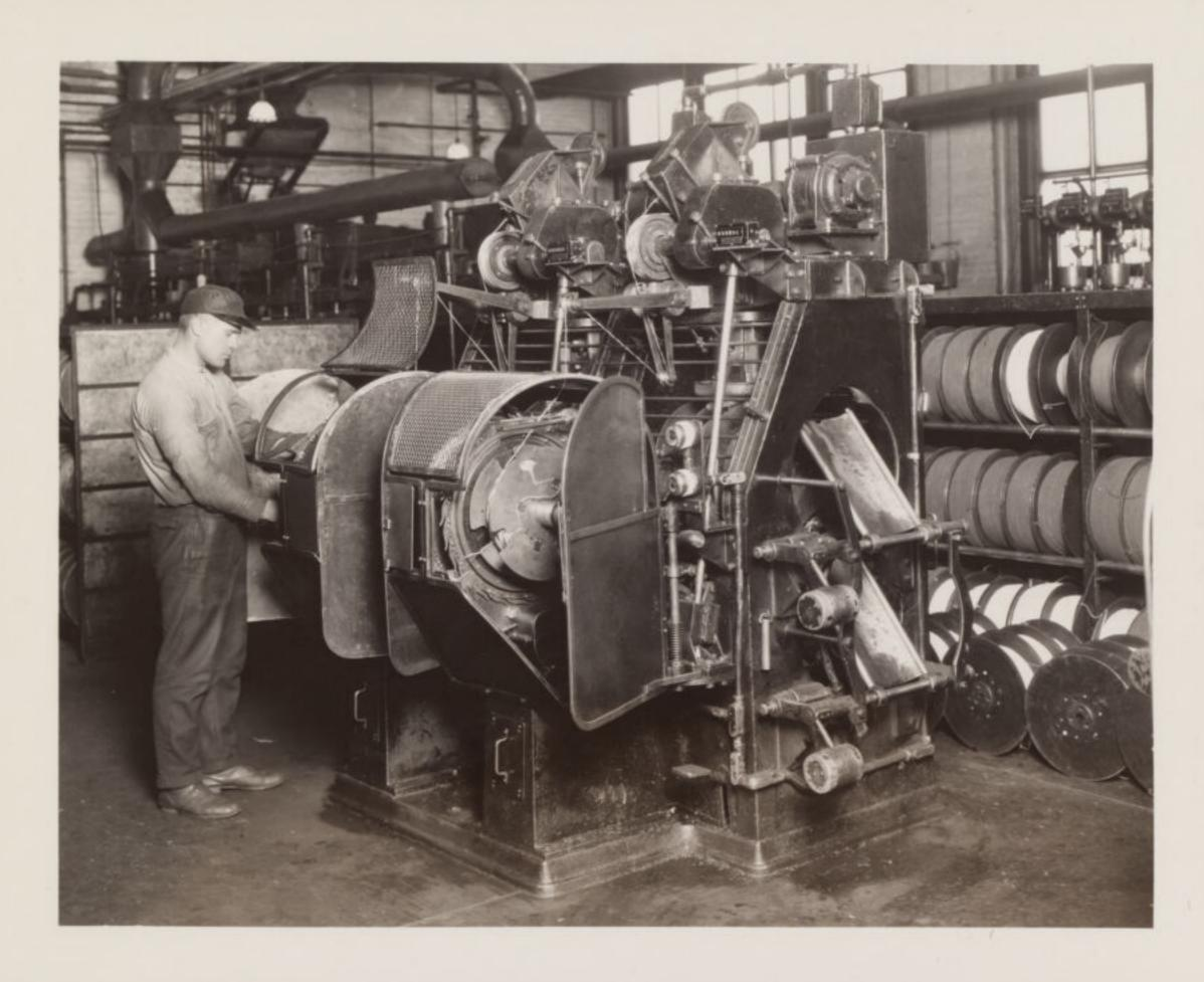
DISTRIBUTING FRAME WIRE TWISTING AND COILING MACHINE
