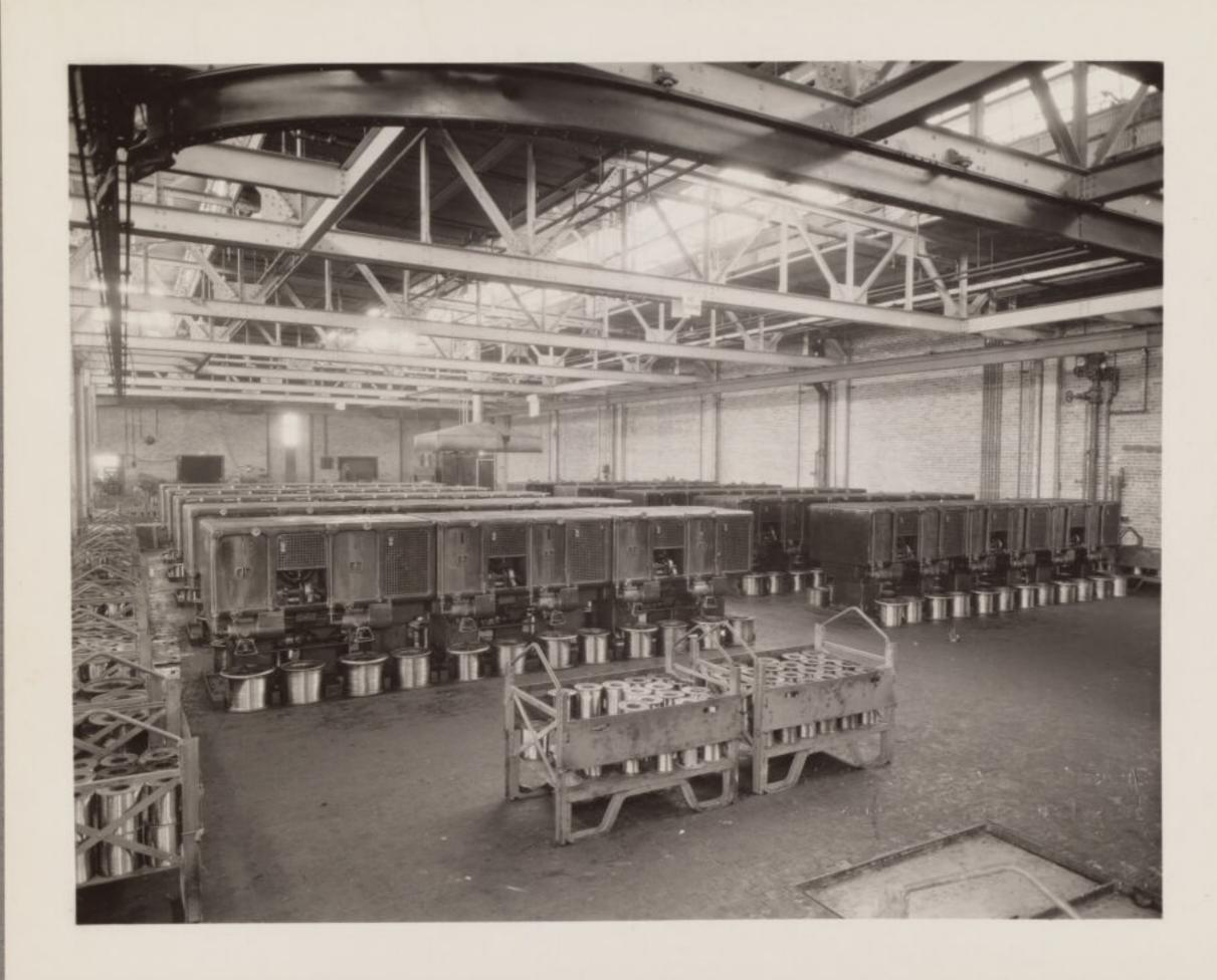
WIRE MILL-INTERMEDIATE AND FINE WIRE DRAWING MACHINES
