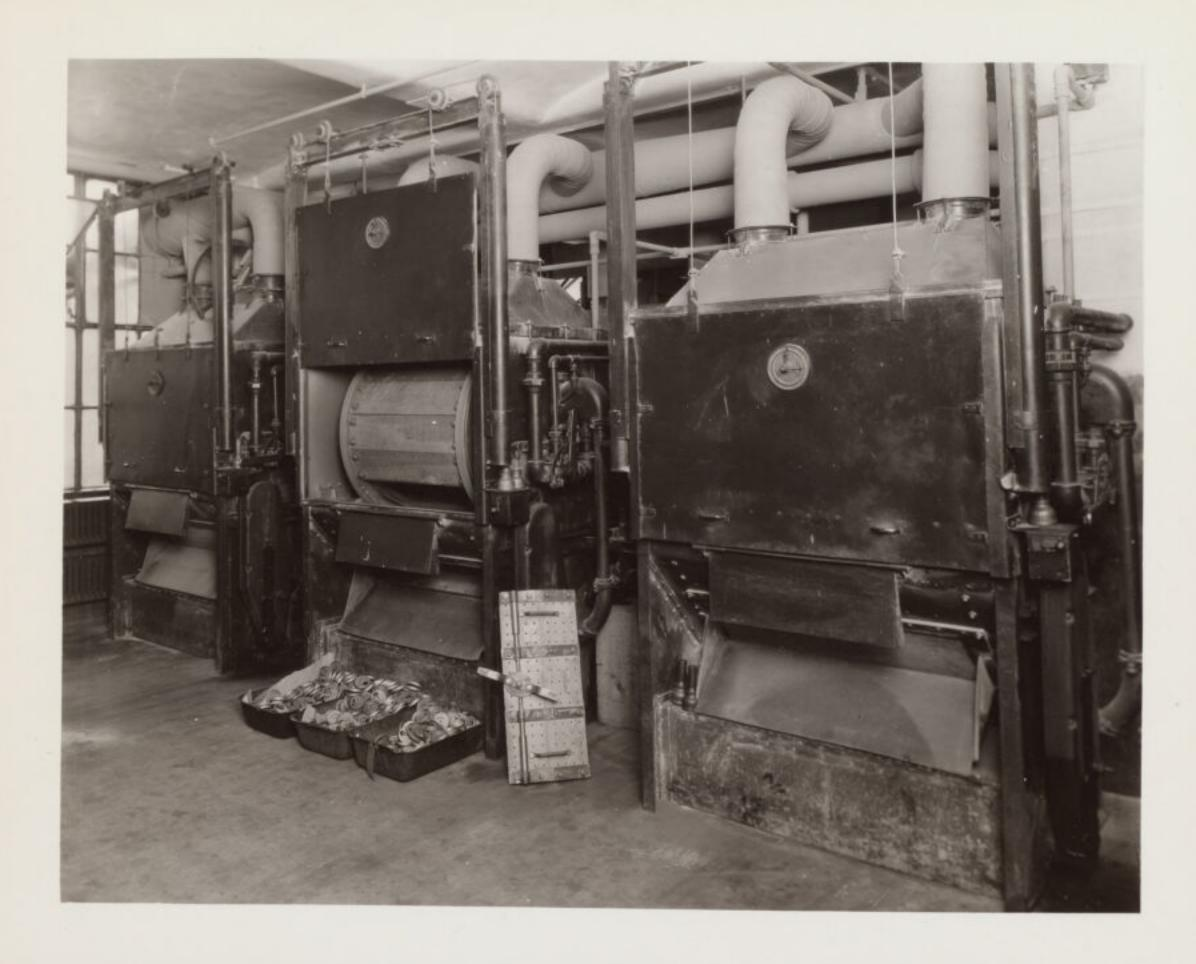
AUTOMATIC BARREL SANDBLASTING EQUIPMENT
